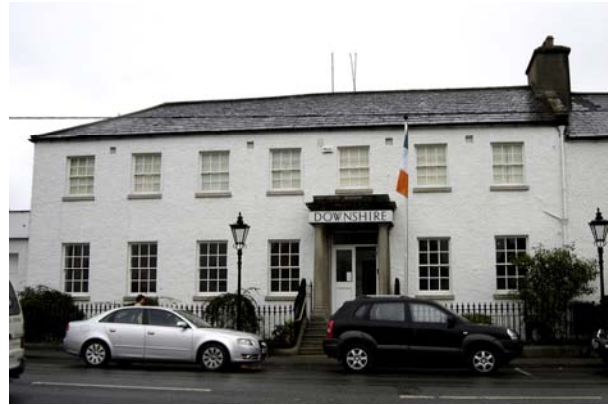
Figure 18 Downshire Arms, Main Street
