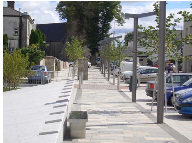
Figure 50 Civic Plaza to the rear of the Town Square, off Main Street
