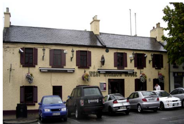
Figure 12 West Wicklow House, Main Street
