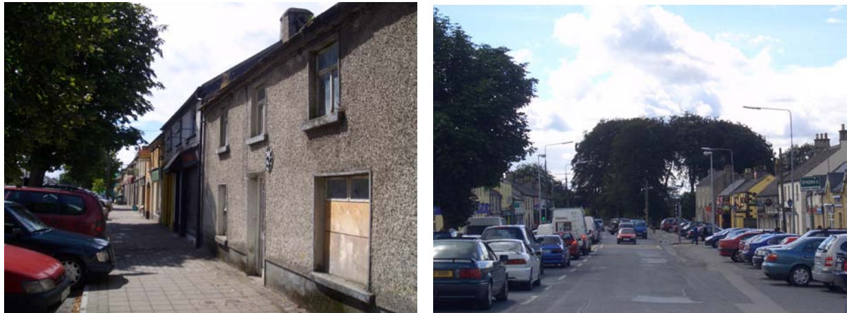
Figure 2 View along Main Street with characteristic terraced streetscape and mature street trees
