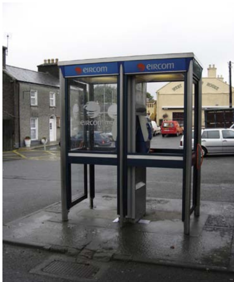
Figure 34 Pair of phone boxes inappropriately located in the Town Square
