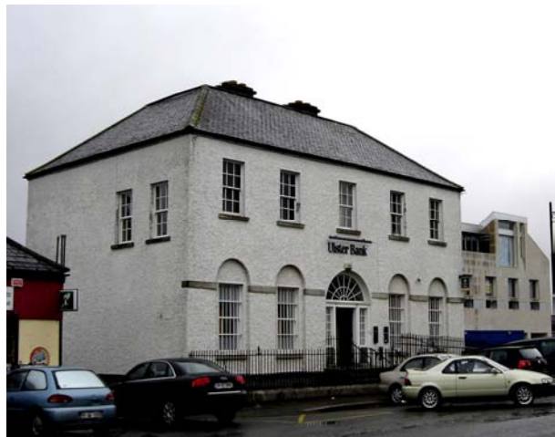
Figure 9 Former Downshire Lodge (Ulster Bank), Main Street
