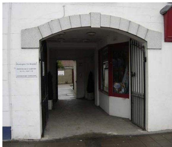
Figure 35 Examples of Carriage Arches on Main Street
