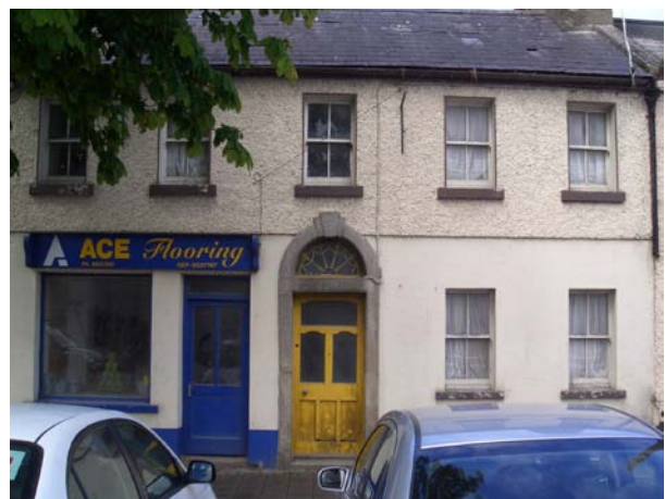
Figure 17 Ace Flooring, Main Street
