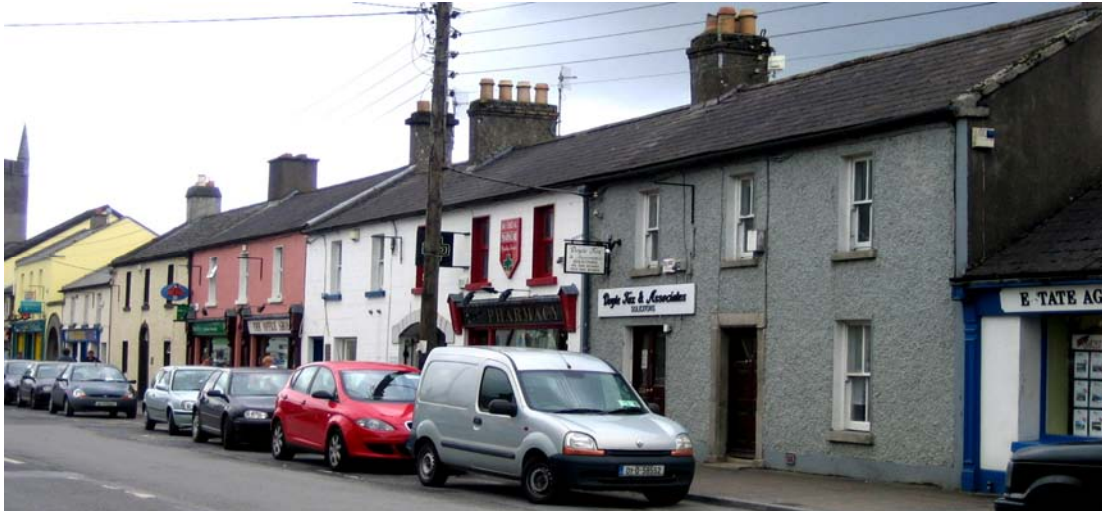
Figure 1 View along Main Street looking northwards (towards Church of Ireland church)
